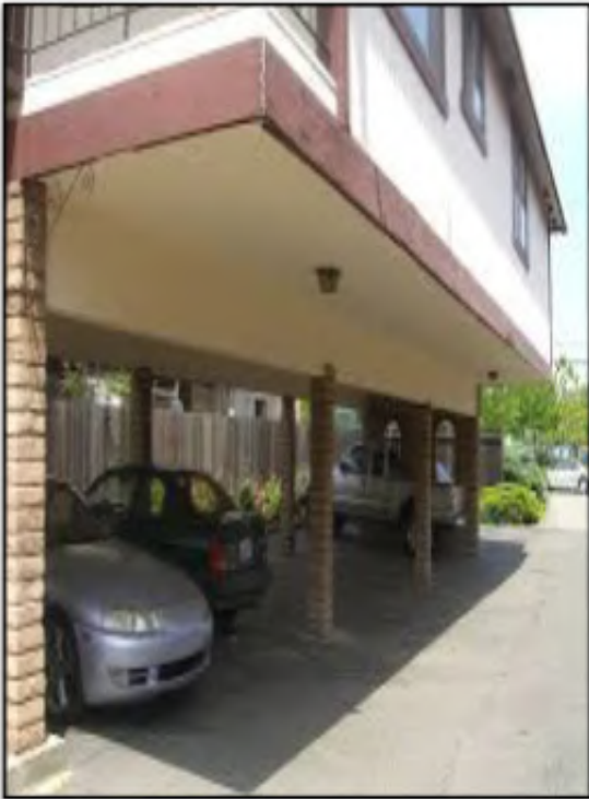
Figure 1: Soft Story for Parking Floor
